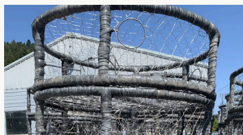
03 Finish Rings fitted, checked
